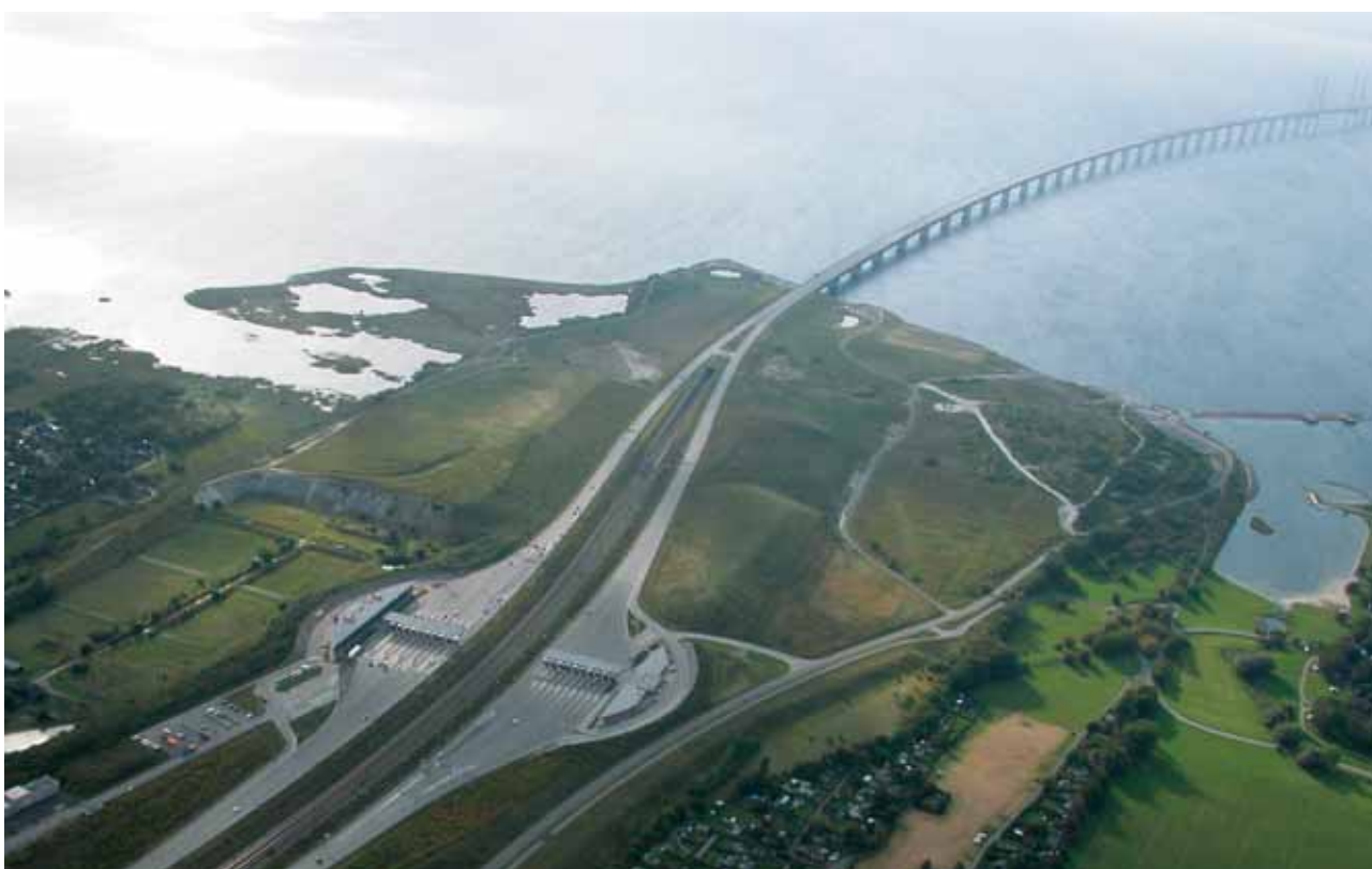
The toll station at Lernacken.
