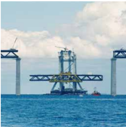
The final bridge span is placed in position.
