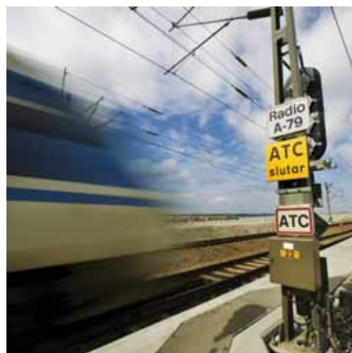
The system border which switches automatically between Danish and Swedish interlocking and ATC systems.
