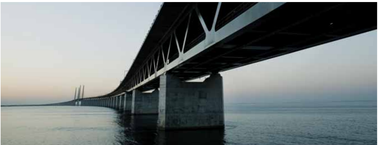
Lower deck of the bridge carrying the trains.
