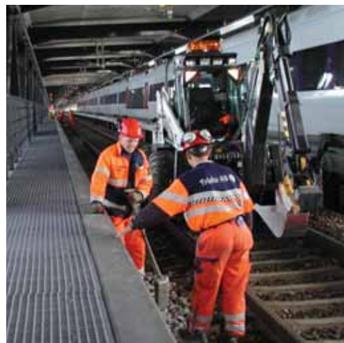
Maintenance of the rail track on the bridge.
