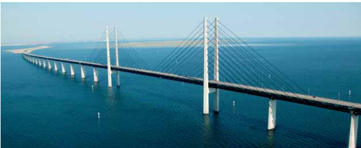
Western approach bridge and high bridge.
